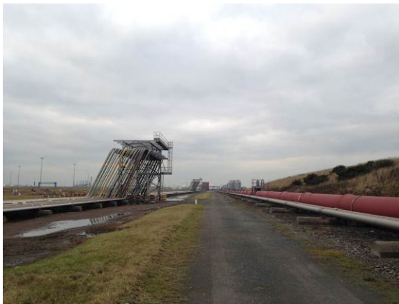
Existing roadway (possible conveyor link)
