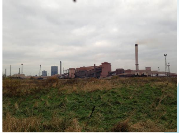
View of Area I site
